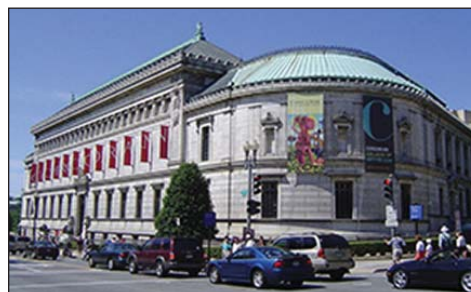
Corcoran Gallery of Art Roof Renovation $8,852,000 | Construction Management at-Risk
