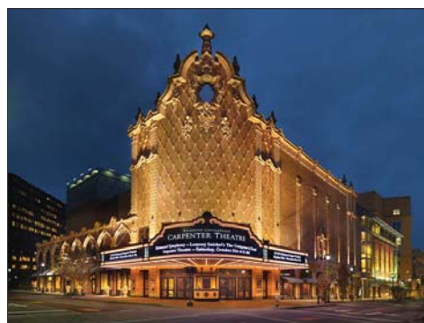
Richmond Center Stage Historic Theatre Renovation $58,300,000 | Construction Management at-Risk
